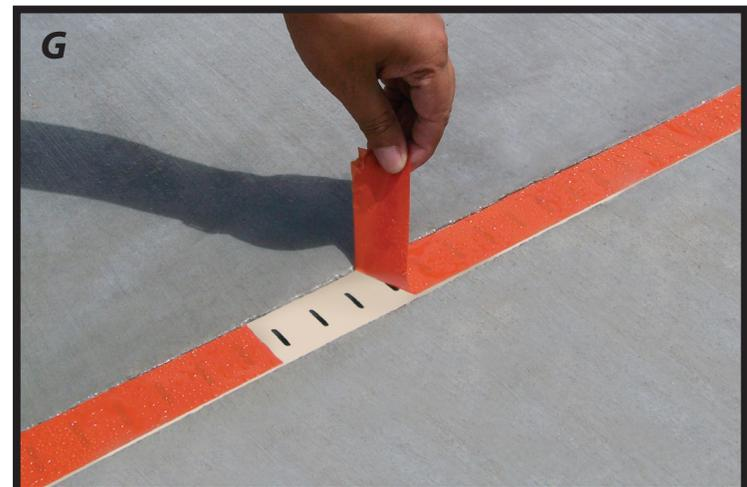
**G.** Remove the protective tape after the concrete installation is complete.
