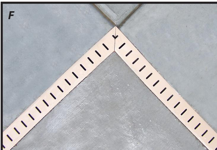
**F.** The fittings (90 degree, 45 degree, etc.) are supplied as "base only". During installation, the top caps (10 ft. long) run continuously over the fittings serving as a mounting device, leaving the fittings virtually invisible.
